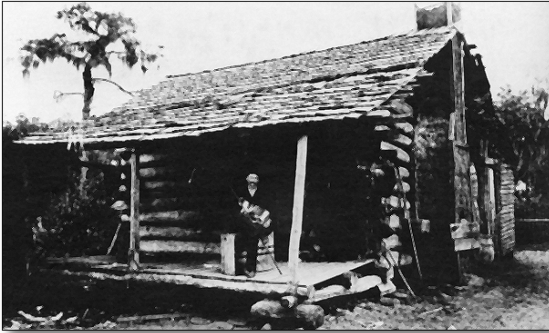
By the 1890s, house styles in Florida varied considerably. This photograph from the Stokes Collection shows a typical “cracker” shanty, built of logs and rough-sawn pine with a mud chimney.
